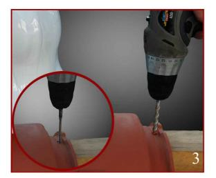
Third, the ridge tile self should be fixed via a countersunk head screw on the dry ridge. For that purpose the nail hole of the ridge tile needs to drilled to be bigger.
