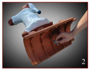
Second, use the included hex bolt and the washer to bolt the figure with the ridge tile together.
